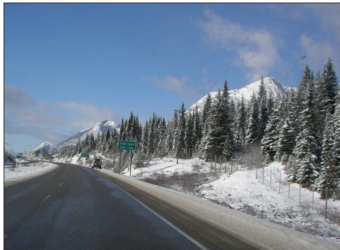
Figure 10. Wildlife exclusion fencing on the Coquihalla Highway.
