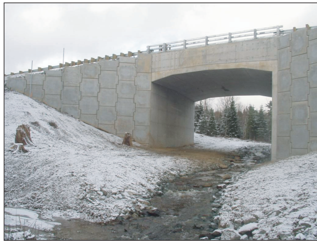
Figure 2. Doyon Creek concrete box culvert before tree and shrub planting.
