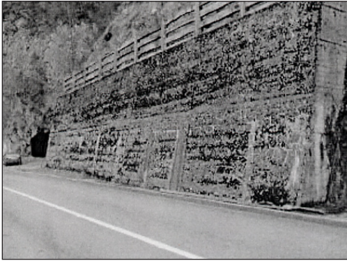
Figure 3. Retaining walls often border close to the roadway, blocking animal movements between habitats on either side of the road.
