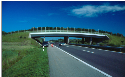
Photo 2. 147.514-km Game Bridge of the M1 Motorway.
