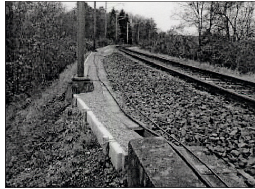
Figure 4. Even low retaining structures can be a strong barrier and prevent free crossing of a structure by small animals. (Photo courtesy to KARCH, Neuchâtel).
