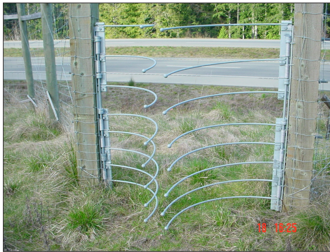
Figure 2. One-way gate designed for moose and deer.
