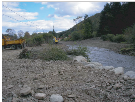
Figure 13. The bench provides an area for high water between the creek and Route 23. The willows were planted and they are doing quite well. The utility pole is not shown but the bench protects it from the creek.
