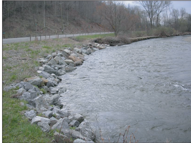
Figure 6. Looking downstream at the bank stabilization installed in 2004 before the June flooding. Route 23 is seen in the photo. Ashcraft Road intersects Route 23 just out of view to the left in the photo.
