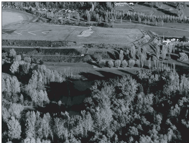
Figure 2. Runways at Seattle-Tacoma International Airport, King County, Washington, are raised above surrounding grade.
