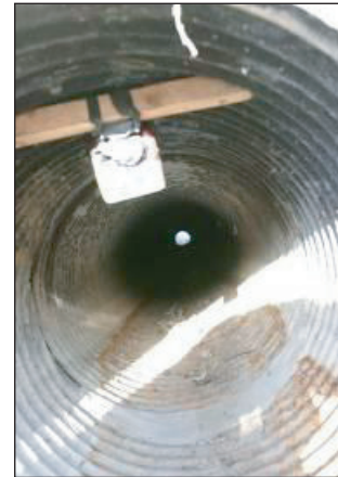
Figure 5. Installed camera in circular culvert
