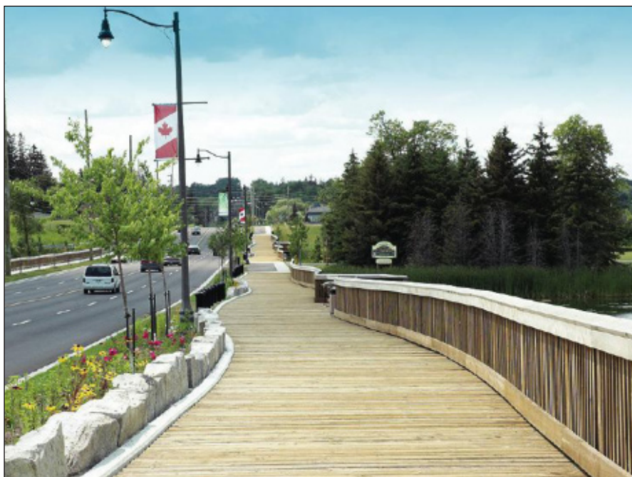
Figure 7. Boardwalk, lighting and viewing platform at the McKenzie Wetland looking west.
