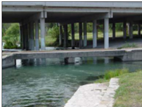
Figure 1. Bedell Street Bridge with U.S. 277 in the background.
