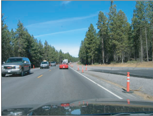
Figure 2. Predicting traffic volume is important when considering terrestrial passage needs within the functional lifespan of a proposed water conveyance structure. Although gravel only few decades ago, this highway has a current ADT at this location of 22,760 and is projected to be 38,700 by 2028 (Oregon DOT). Photo S. Jacobson.
