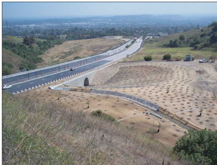
Figure 1. Completed underpass at Harbor Boulevard located in the City of La Habra Heights (Los Angeles County) May 2006.
