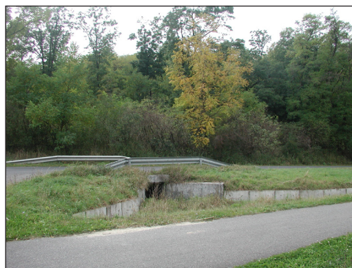
Photo 4. Sophisticated amphibian tunnel system.
