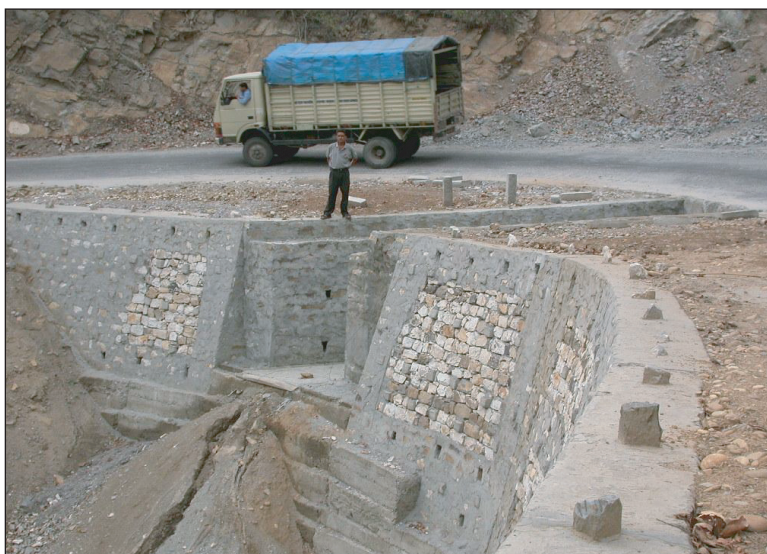
Figure 7. Construction of big culvert and check dam for proper drainage throughout the length of the road passing along the Upper Ganges.
