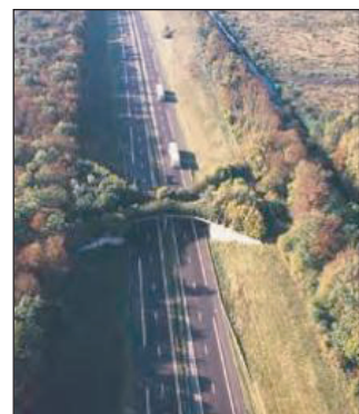
Fig. 4. 3 rd generation of fauna passages. Parabolic shape at the A36. (Source: SETRA and CETE, 2006)
