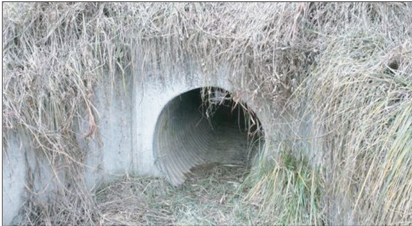
Figure 4. Circular culvert (waved steel pipe)
