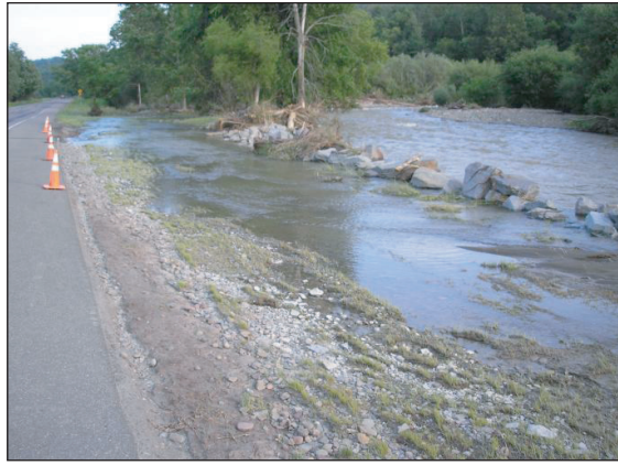
Figure 8. Canasawacta Creek is undermining Route 23. This is where the creek was moved from the north side of the road to its present location. Flooding occurs often in this location.
