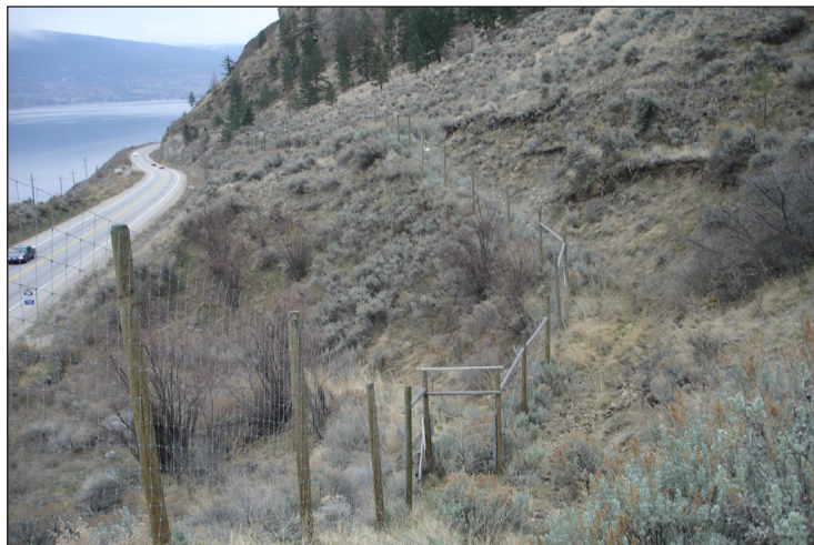
Figure 14. Highway 97 between Peachland and Summerland.
