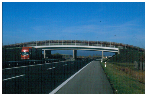
Photo 3. 151.709-km Game Bridge of the M1 Motorway
