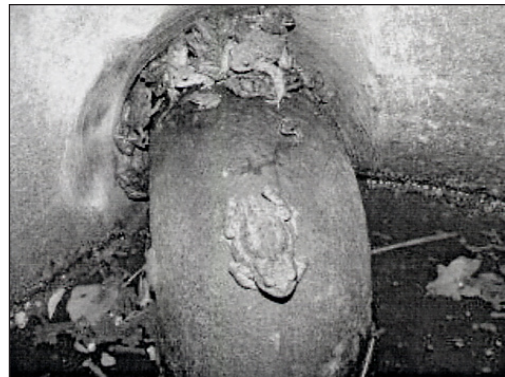
Figure 6. With no direct exit possibility, trapped toads and frogs either die in the chute or will, in the course of the next rain storm, get flushed into the sewer system via the siphon. (Photo courtesy to Amphibtec, Gelfingen)
