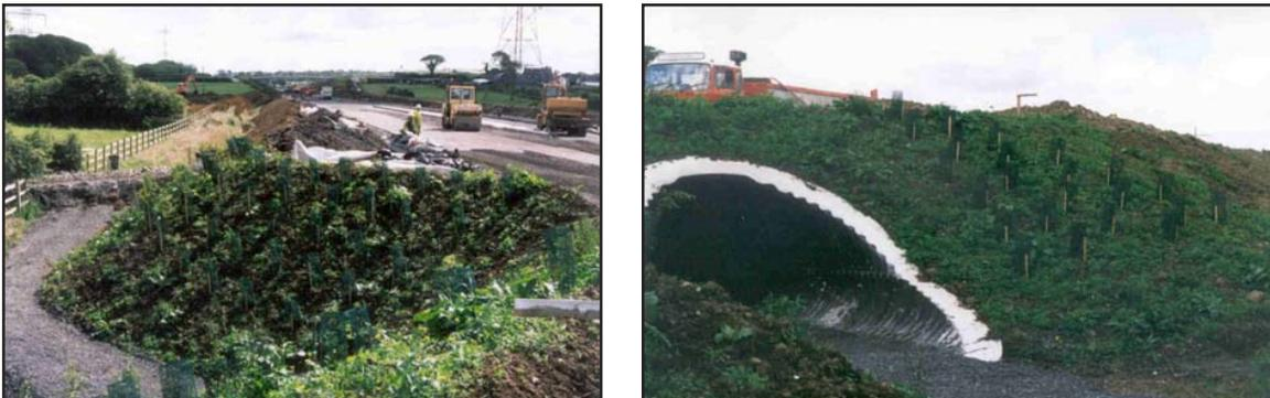
Figure 3. Planting at the bat culvert. These photographs show the planting at an early stage. In the photograph to the left, the culvert is located in the recess.
