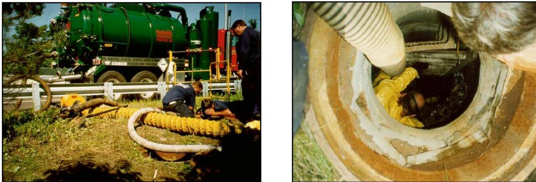
Figure 3. Vacuum truck employed during the cleaning operation of a water-quality inlet along the Southeast Expressway in Boston (left) and a maintenance worker pushing sediments to a vacuum hose while exercising “confined-space entry” protocol (right).
