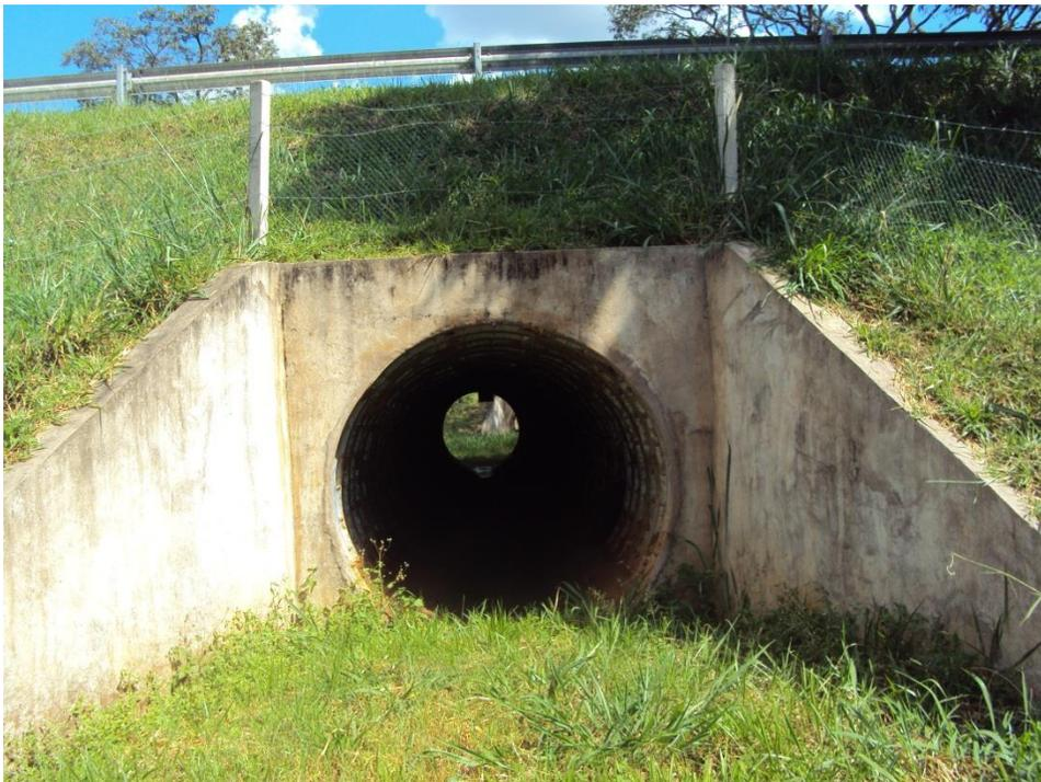
**FIGURE 2.** An example of a 1.7m diameter culvert under a highway evaluated for the cost-benefit analyses (Copyright © 2012, by Fernanda D. Abra).
