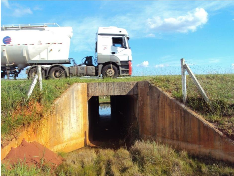
**FIGURE 3.** An example of a box culvert under a highway evaluated for the cost-benefit analyses (Copyright © 2012, by Fernanda D. Abra). Note that this particular culvert measures 2.00x2.00m and that we evaluated a culvert that is 3.00x3.00m.
