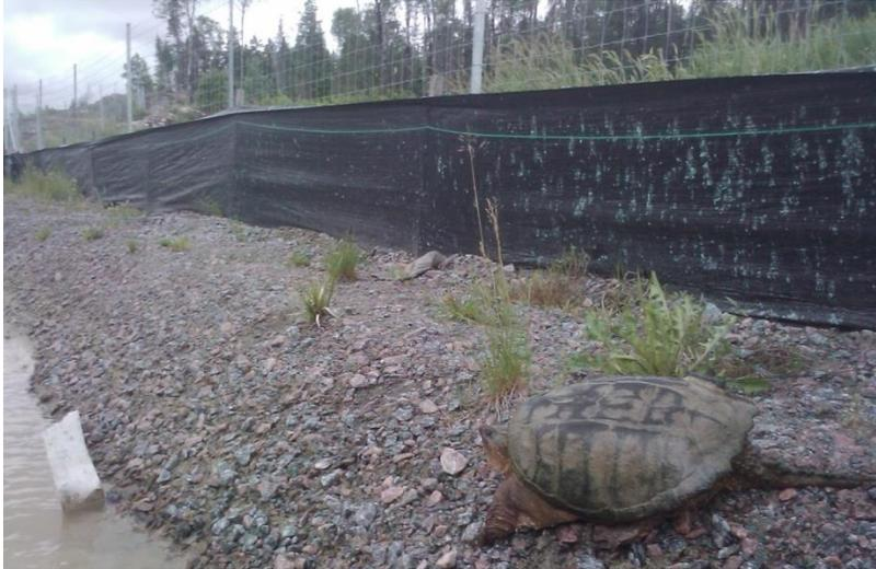
**FIGURE 1** The reptile fence (0.8 m tall), affixed to a large mammal exclusion fence and buried at the base (0.2 m deep). A female snapping turtle navigates along the fence in an effort to find a gap to reach the wetland-side after becoming trapped on the traffic-side of the fence during a nesting season movement.
