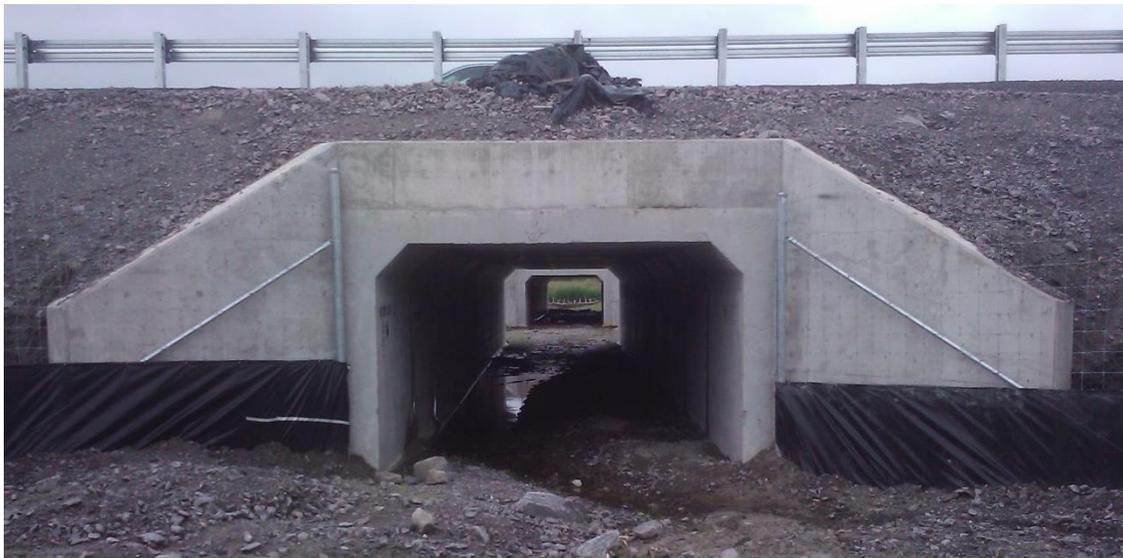
**FIGURE 2** The ecopassage running below the north bound (foreground) and south bound (background) lane of Highway 69 near Shepard Lake, Ontario; a large 15.25 m gap between the culverts allows for increased light with the ecopassage.
