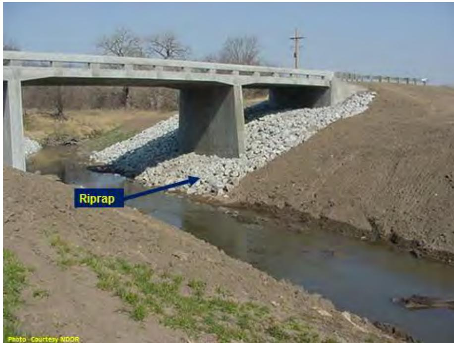
**FIGURE 1. Typical scour protection on Nebraska bridges.**
