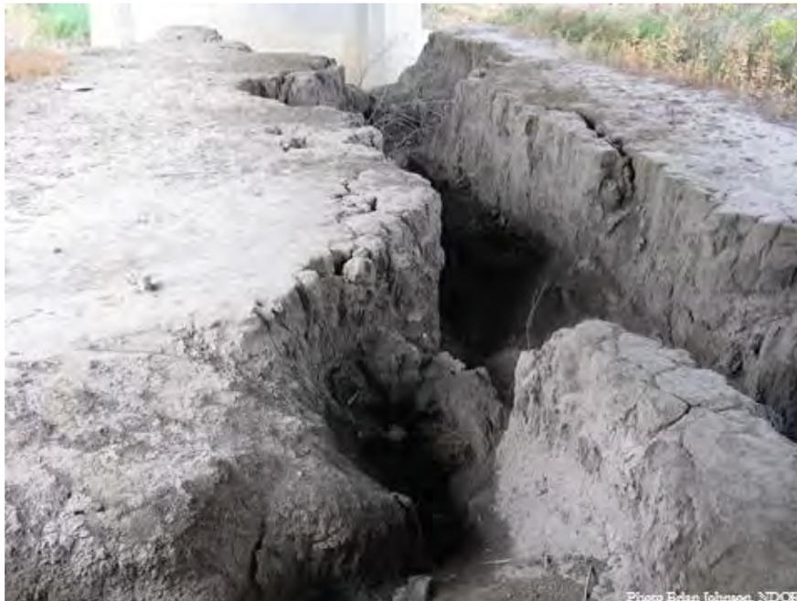
**FIGURE 8. Example of the erosion that can occur along the drip line of an unprotected undercrossing. Salt Creek Bridge, Mile Marker 407.97, October 2010.**
