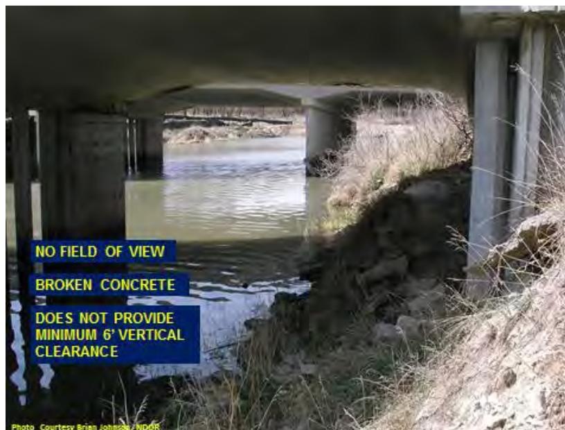
**FIGURE 6. Existing Sarpy Ditch Bridge undercrossing.**
