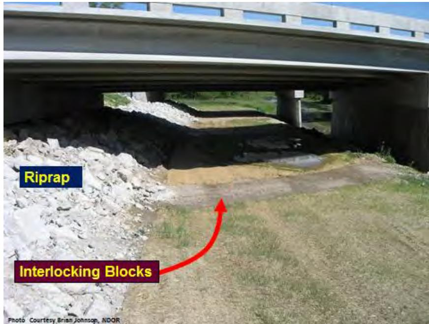
**FIGURE 7. New wildlife undercrossing at Sarpy Ditch Bridge, May 2009.**
