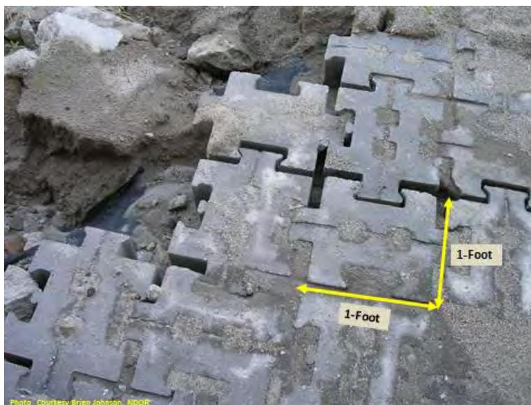
**FIGURE 2. Interlocking pavement blocks.**
