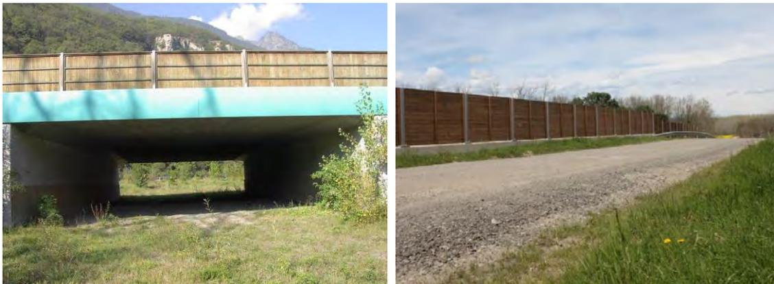
**Figure 6. Wildlife crossings could be specific for wildlife (underpass, left) or multifunctional, created by adapting existing structures (overpass, right).**
