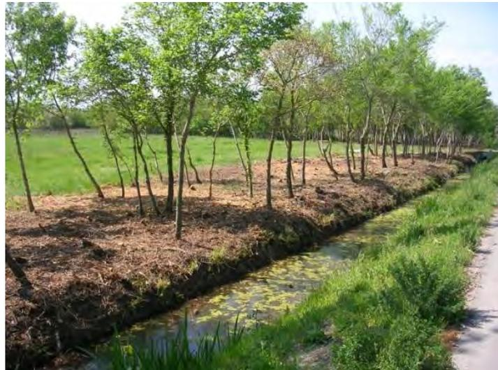
**Figure 8. Verge management consists of cutting existing vegetation and eliminating animal refuges in a 3-m strip along both sides of the road.**
