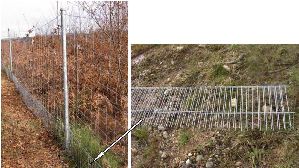
**Figure 5. On stretches with fences that are not buried, specific reinforcements can be added to the bottom of the fences to prevent wild boar entrance.**
