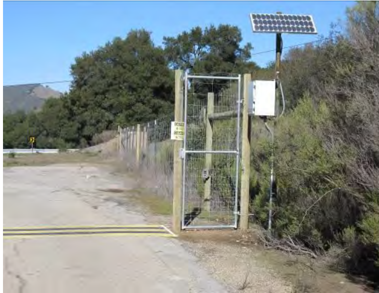
FIGURE 5 Electric mat and solar panel.
