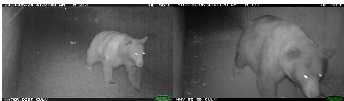
FIGURE 11 Black bear using 4x8 ft. (left) and 4x4 ft. (right) box culvert.
