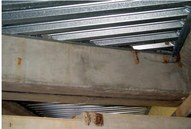
**FIGURE 6 Staining of crevices and transverse beam by guano and urine under bridge in Lamar County.**
