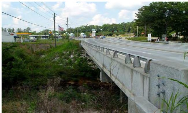
**FIGURE 13 Bridge with ends blocked by vegetation, access at bridge center.**
