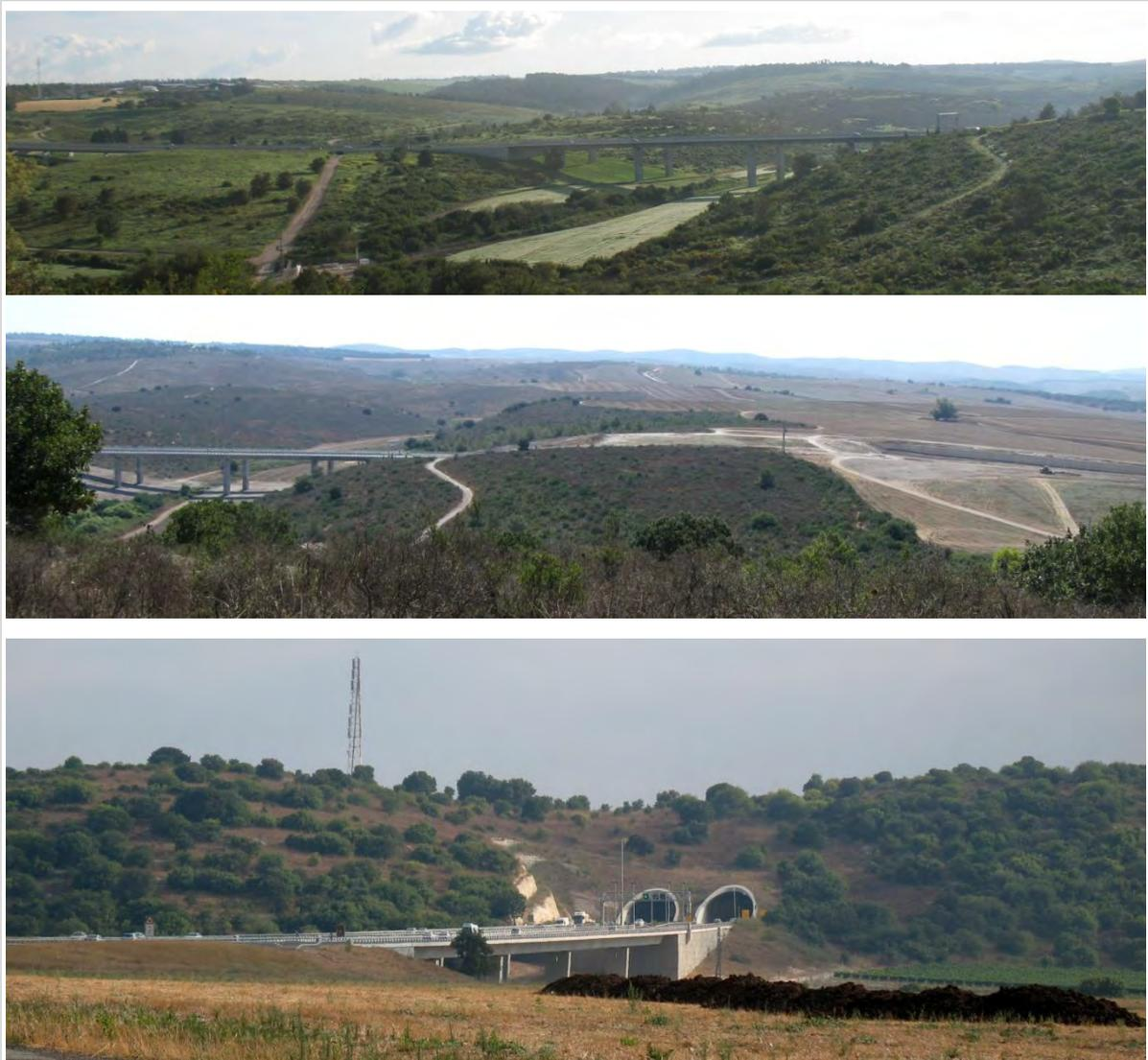
**FIGURE 3 Two of the long bridges (top), the bridge linked to the cut & cover ecoduct (middle), the tunnel ecoduct (bottom).**
