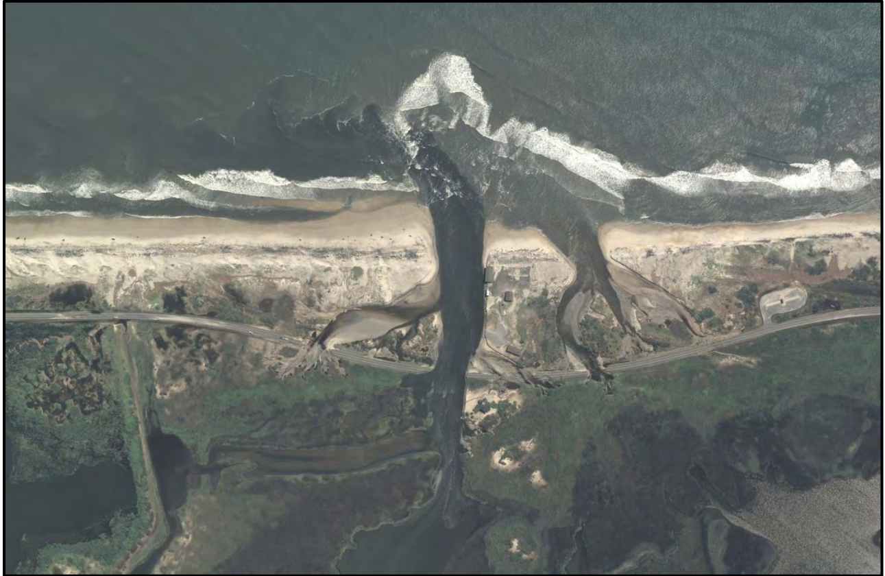
FIGURE 3 Aerial photo of Pea Island Inlet taken August 28, 2011: one day after Hurricane Irene. The breach in NC 12 can be seen in the middle.
