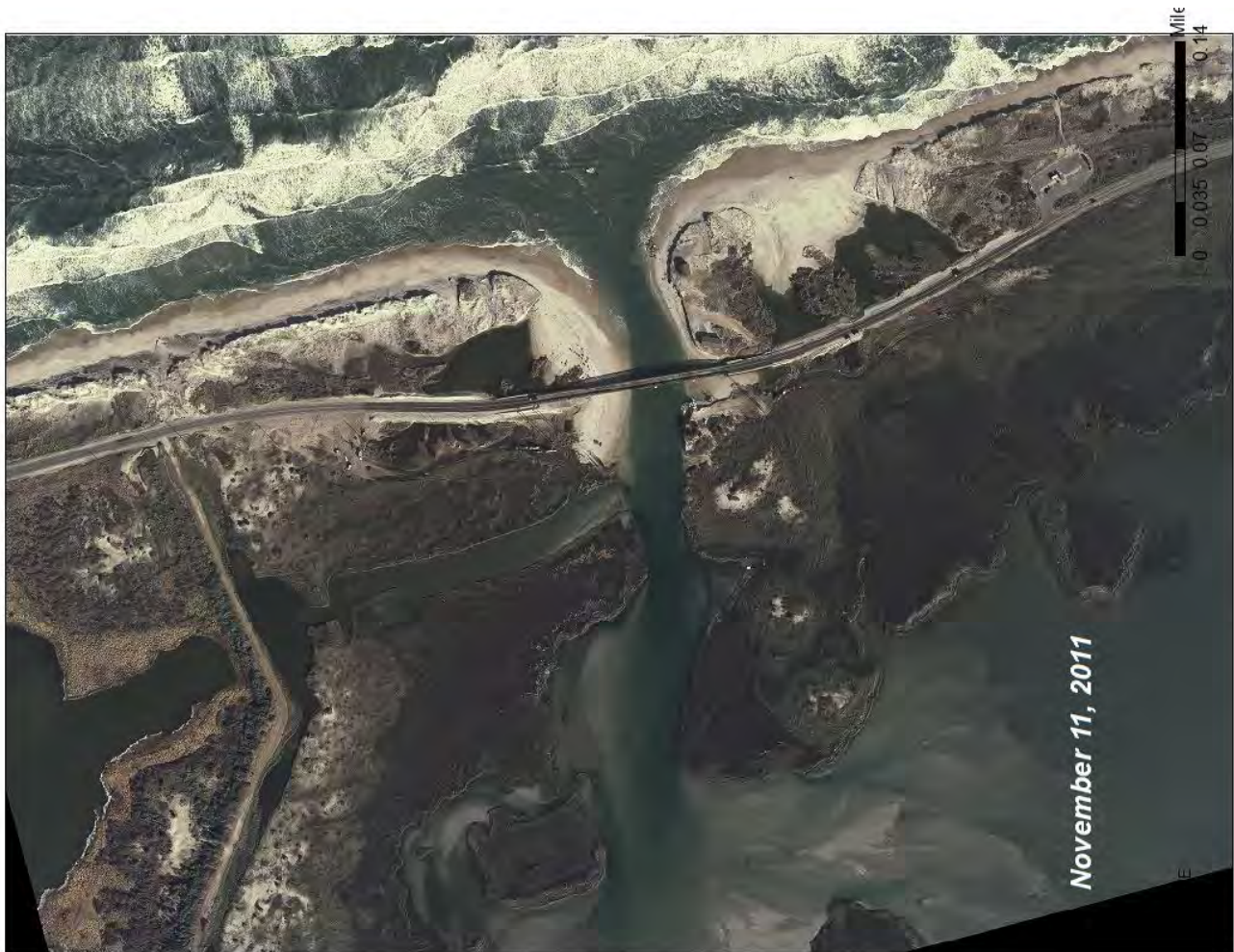
Figure 5 Bridge over Pea Island Inlet
