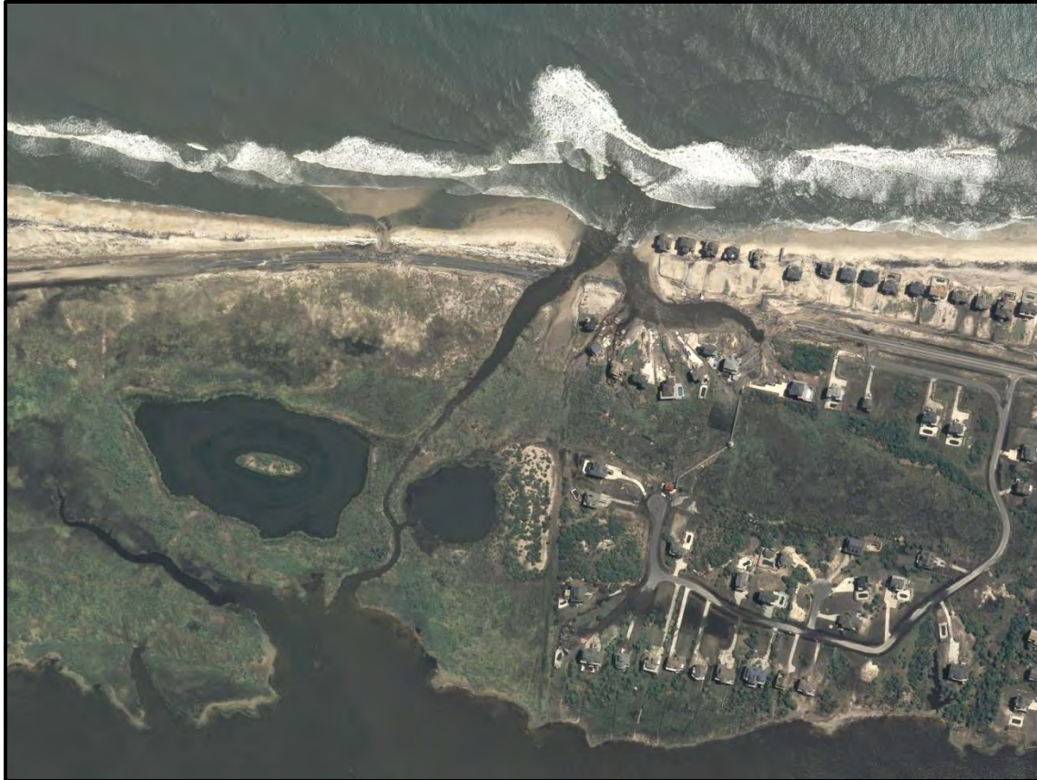
FIGURE 4 Ariel photo of the breach at Rodanthe "S Curves" taken August 28, 2011.
