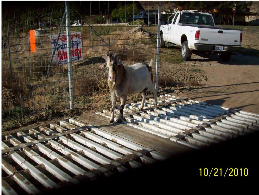
**FIGURE 2. Pet goat easily crosses a first generation wildlife guard, designed to accommodate a snow plow blade**
