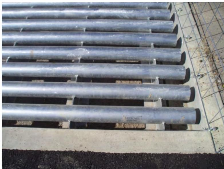
**FIGURE 3. WSDOT's final wildlife guard design employed round pipe for cross pieces.**
