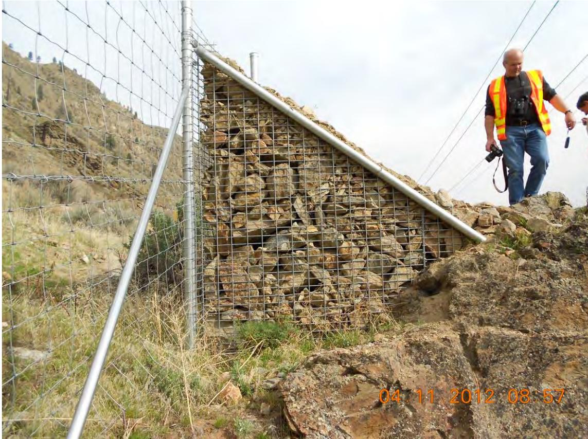
**FIGURE 4. Jumpout designed for bighorn sheep was placed atop a rock outcrop.**
