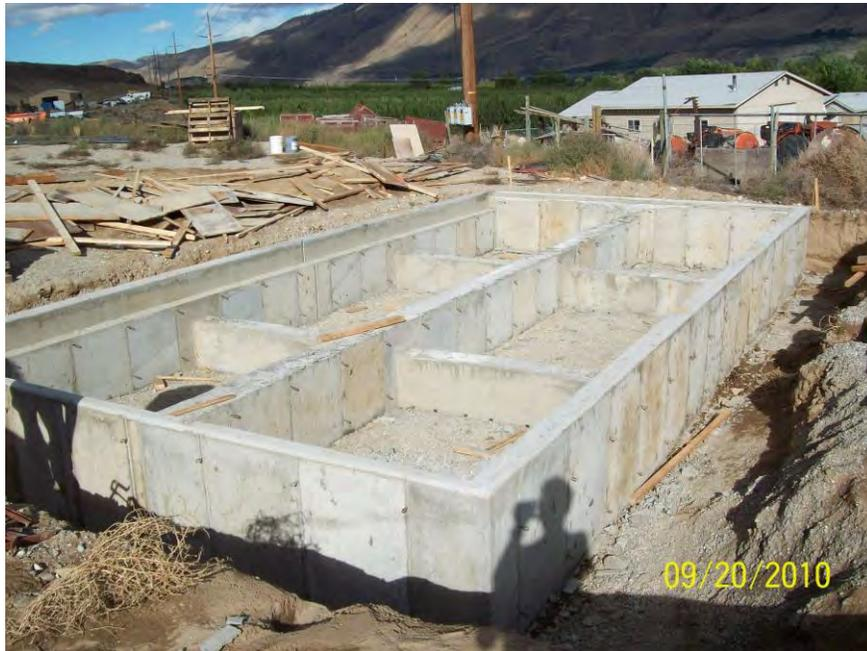
**FIGURE 1. Custom designed foundation for one of ten wildlife guards built for the project**
