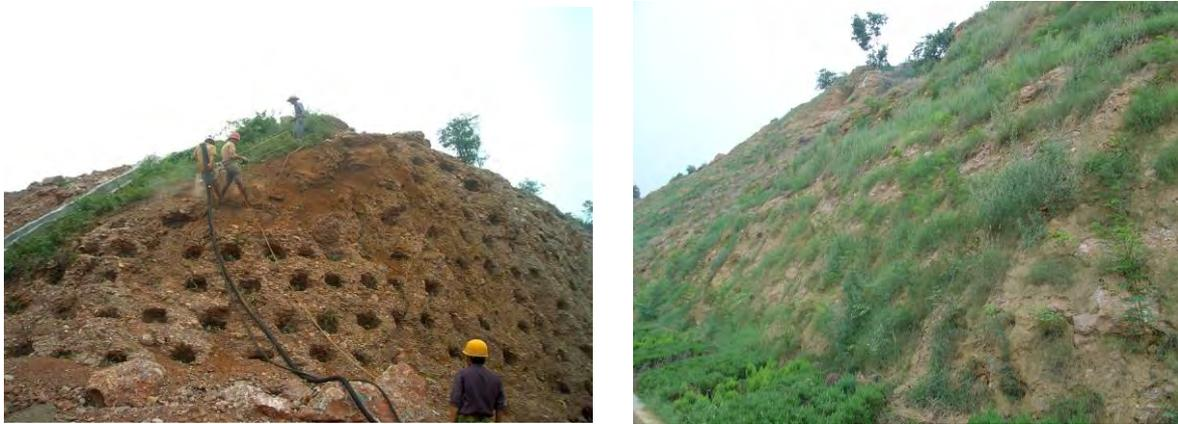
**FIGURE 10 Digging hole and filling soil for greening. left: before seeding, right: after seeding**
