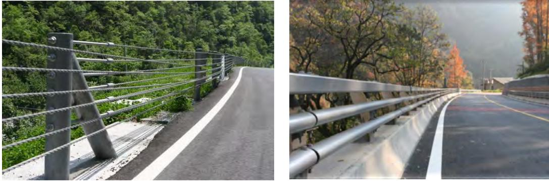
**FIGURE 5** The cable safety fence (left) and the steel safety fence (right)
