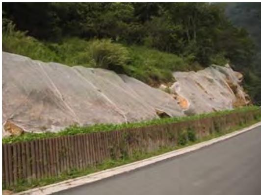
**FIGURE 3** The trunks of cut tree were used to build retaining walls
