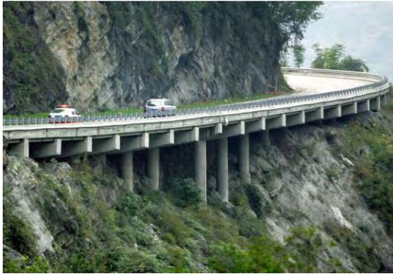
**FIGURE 1** Half-width bridge and half-width previous roadbed
