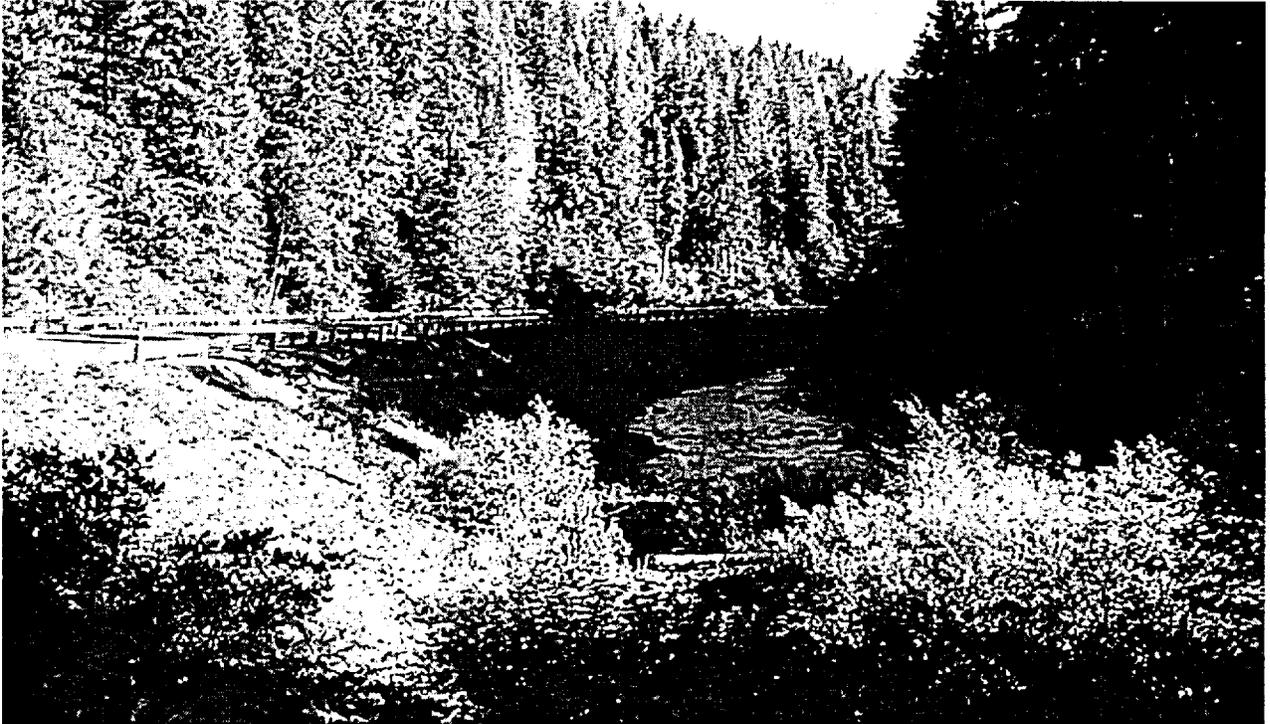
Figure 4. Relocated channel of the North Santiam River along Highway 22, Oregon. Channel has been confined against the hillslope (right). Old cut-off river bends are still existing to the east (left) of the highway.
