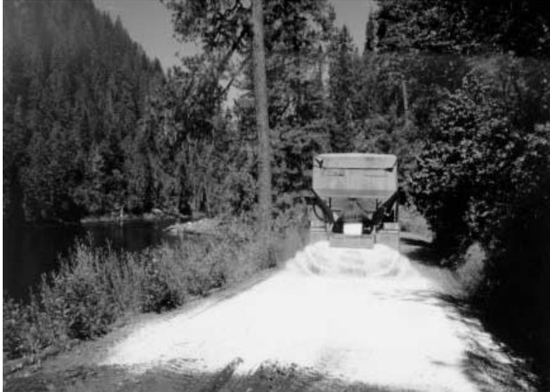
Fig. 5. Calibrated spreader applying Calcium Chloride to a previously processed road. The result is a finished road with a hard, smooth, maintainable driving surface. Grinding with the In Place Processor also works well in frozen soil, as the rocks stay in place for crushing. Some dampness in the soil is preferred for decreased machinewear, dust control, and compaction.
