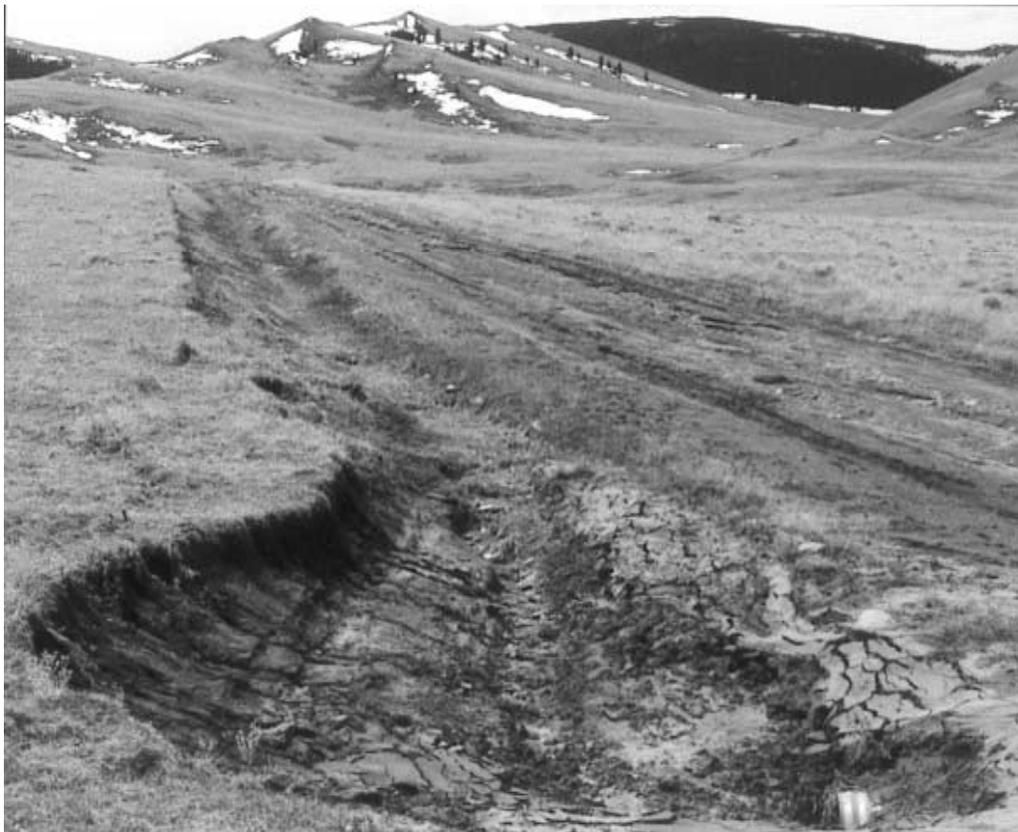
Fig. 2. Road damage resulting from lack of maintenance.
