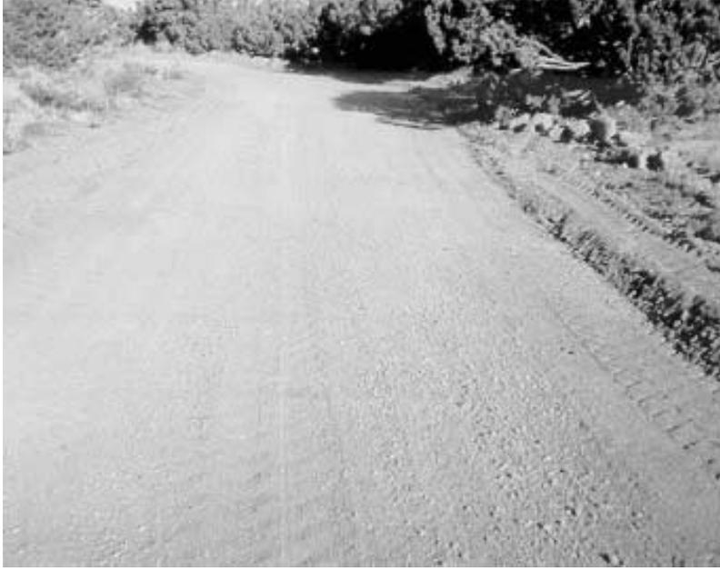
Fig. 7. A typical road section after in-place processing.
