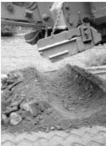
Fig. 4. Rotary drum processing a road surface.
