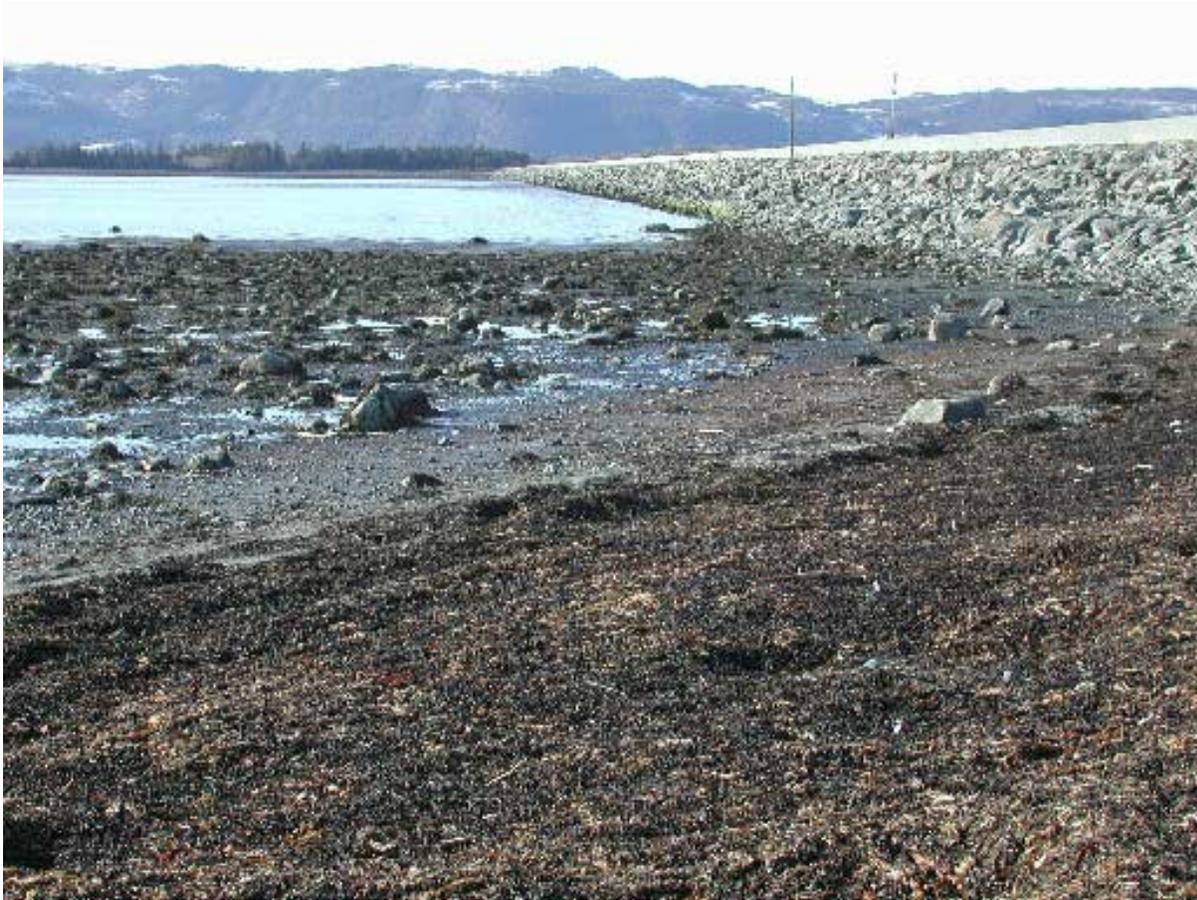
Fig. 5. At low tide, shore areas are exposed on both sides of the embankment, thus allowing animals free passage. This presents a challenge when it comes to finding a wildlife deterrent method that blends in with the natural environment. (Photo: Bjørn luell)
